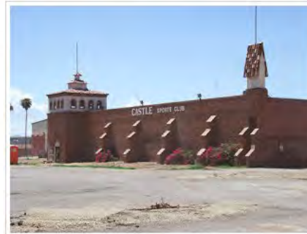
El Cid Castle before its demolition. Photo by: Tony the Marine
